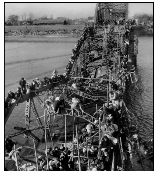
North Korean Refugees Crossing Damaged Bridge
